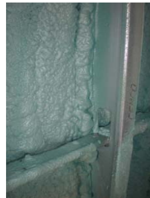
Spray foam insulation
