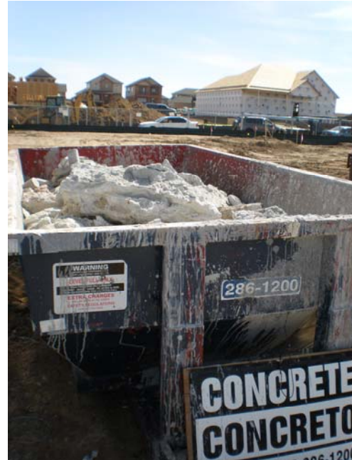
Concrete collection dumpster
