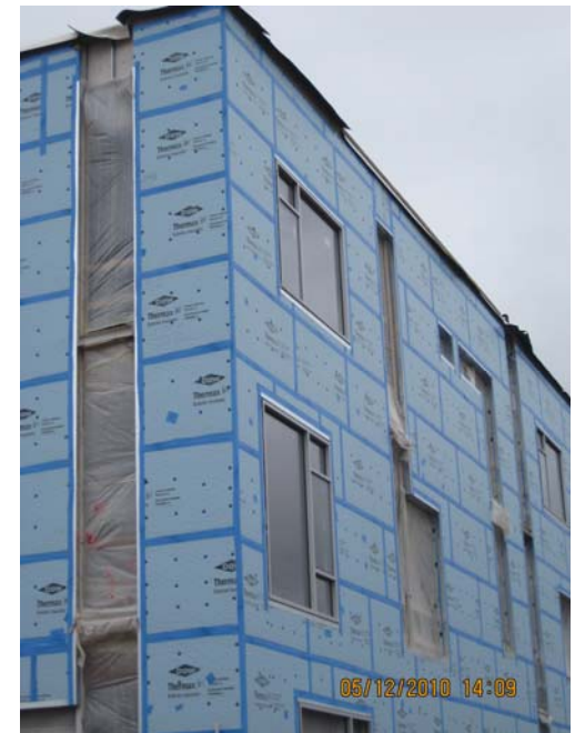
Thermax rigid insulation
