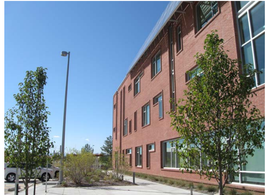
Locally sourced brick
