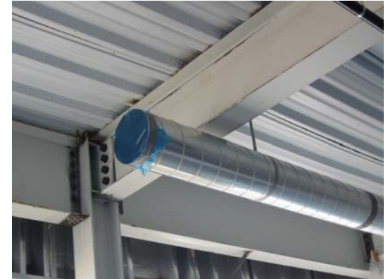
Ducts protected with plastic during construction
