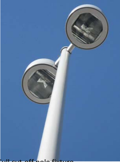
Full cut-off pole fixture
