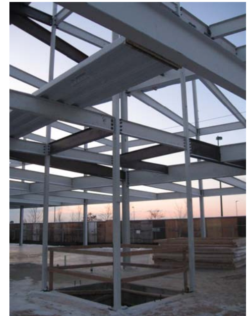
Steel building structure
