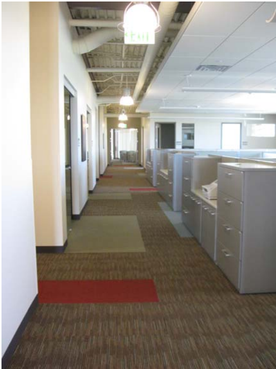
The carpet, gypsum board and ceiling tiles all have recycled content
