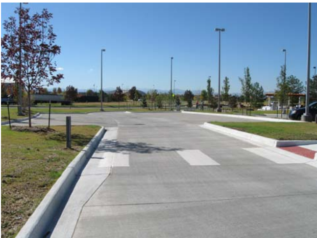
Parking lot with concrete paving
