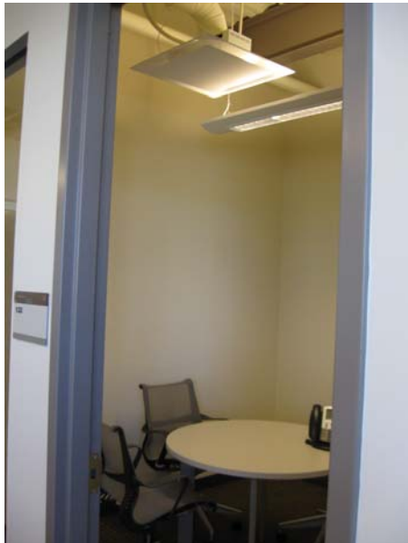
Duct with Thermafuser
